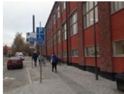
D - Bad ground floor - Major physical investment needed
