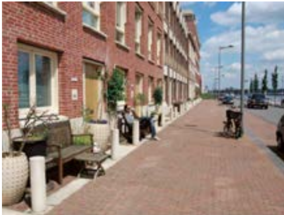
Residential ground floors
