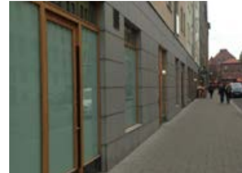
B - Ground floor with potential - Good physical structure - Use improvement needed
